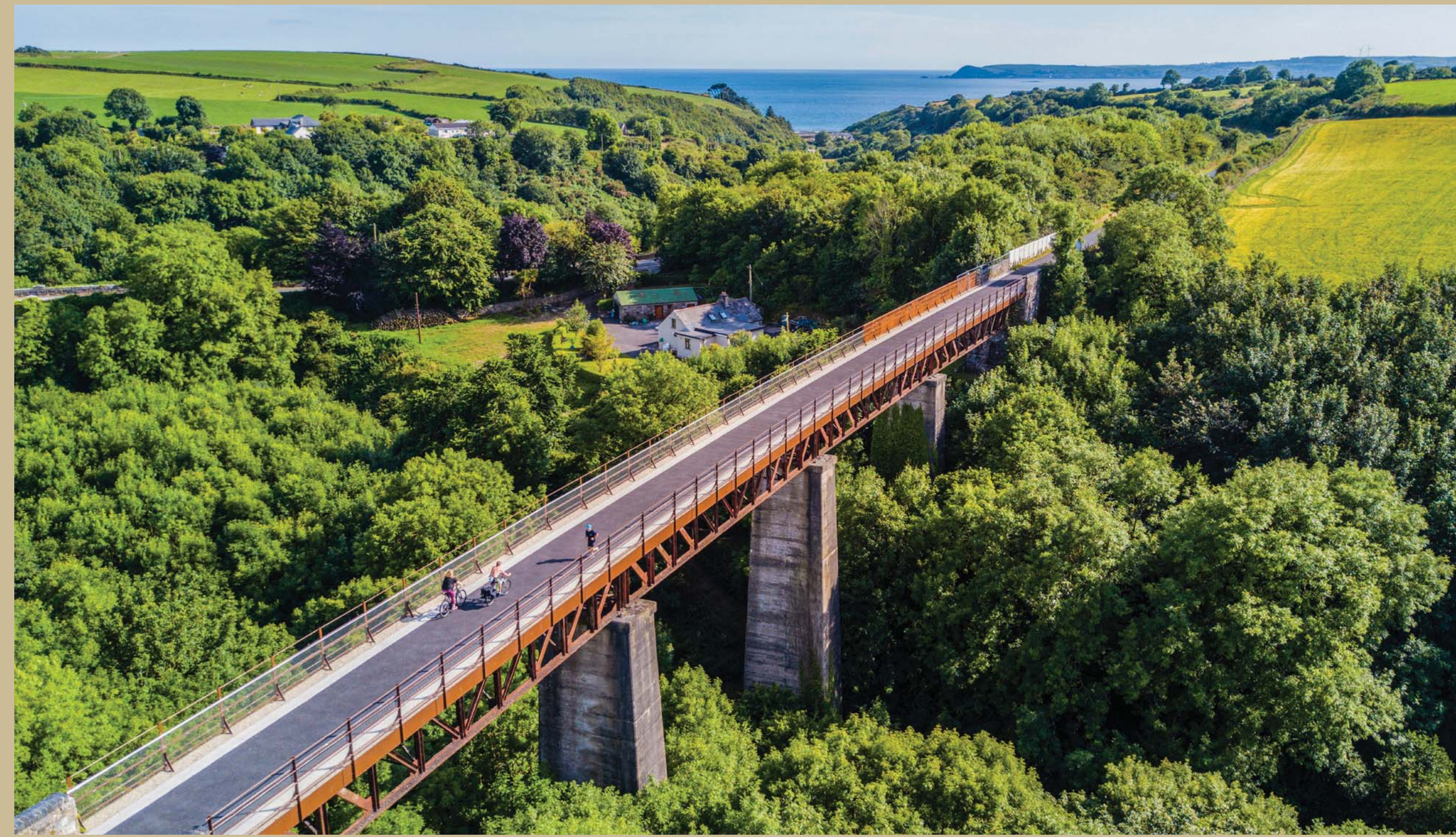
Ballyvoile Viaduct on the Waterford Greenway, (Waterford City and County Archives) Tarbhealach Bhaile Uí Bhaill ar Ghlashealach Phort Láirge (Cartlanna Chathair agus Chontae Phort Láirge)
